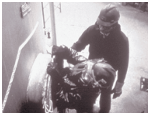
A worker crosses the plane of entry into a confined space.
